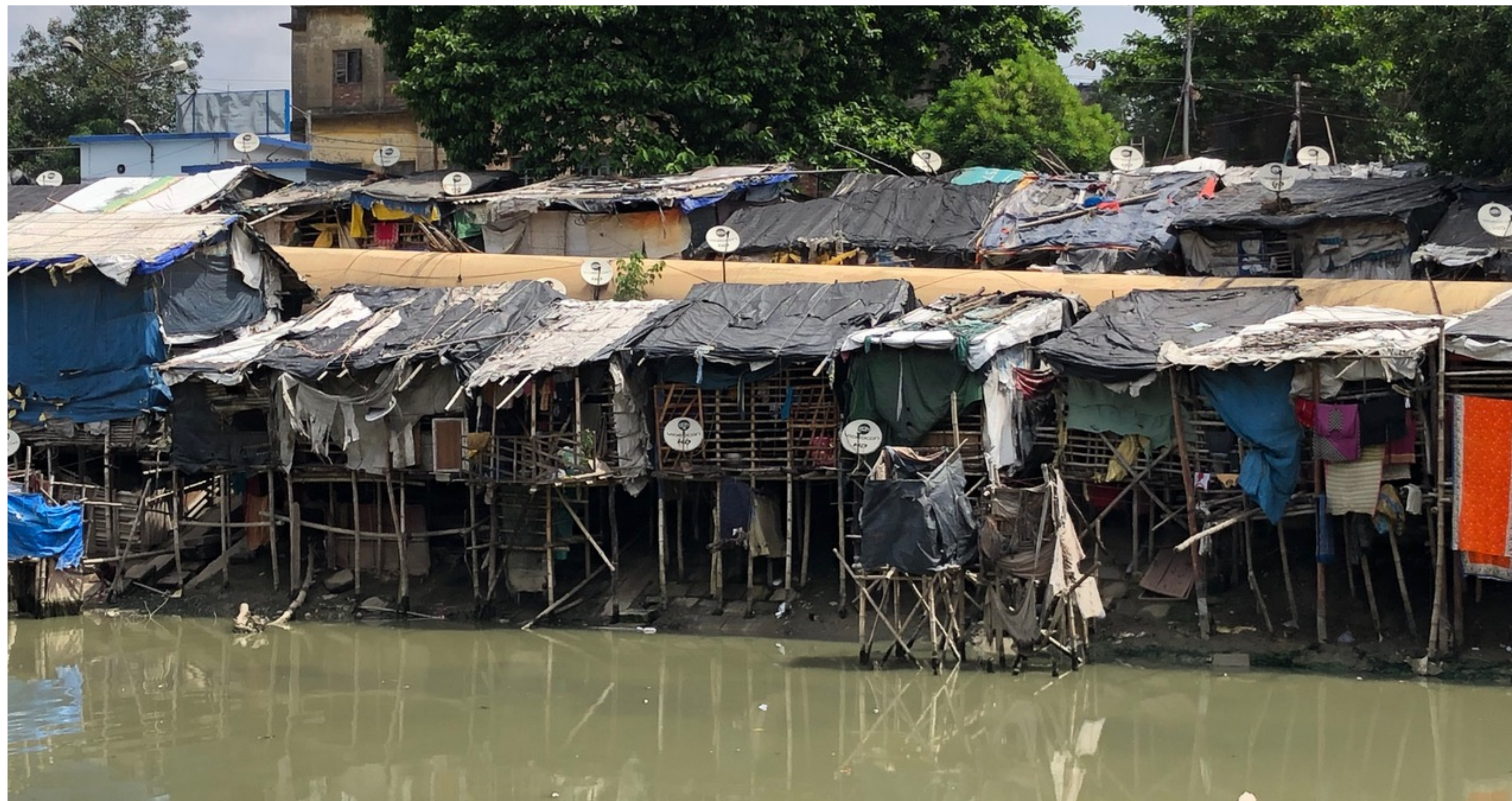
Slum dwellings along the canal are highly vulnerable to flooding
